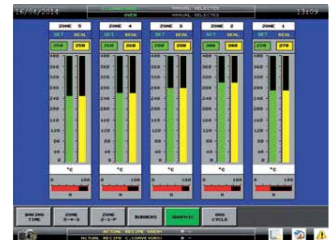
HMI panel displays the programmed, and actual temperatures of each oven zone, using a bar graph-type display, which makes it easy to compare and adjust settings if required
